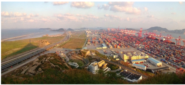
Fig. 10 Shanghai Shengdong International Container Terminal (SSICT)
